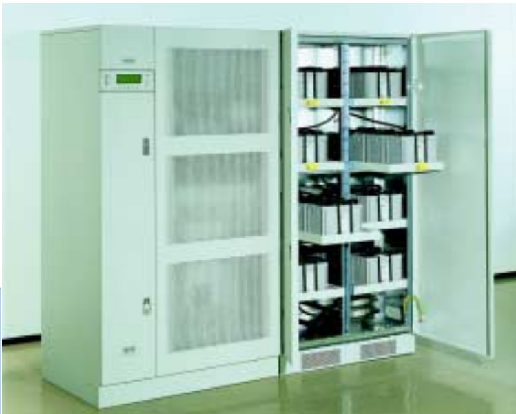
UPS with battery cabinet
